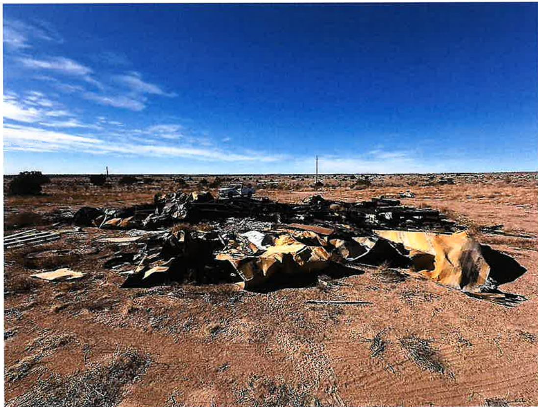
Photo 60. Burned structure in subject property, east of 20 th St NW, looking southwest
