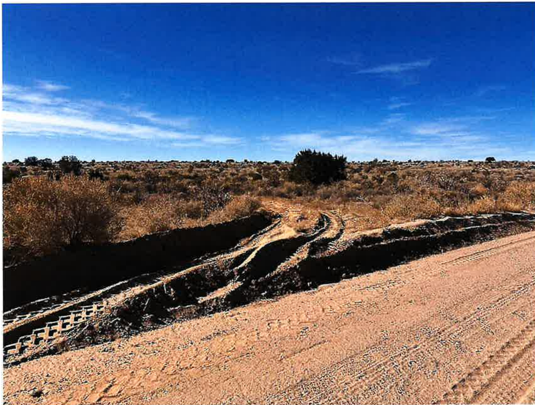
Photo 62. Erosion control along northern boundary of subject property, looking southwest along King Blvd NW
